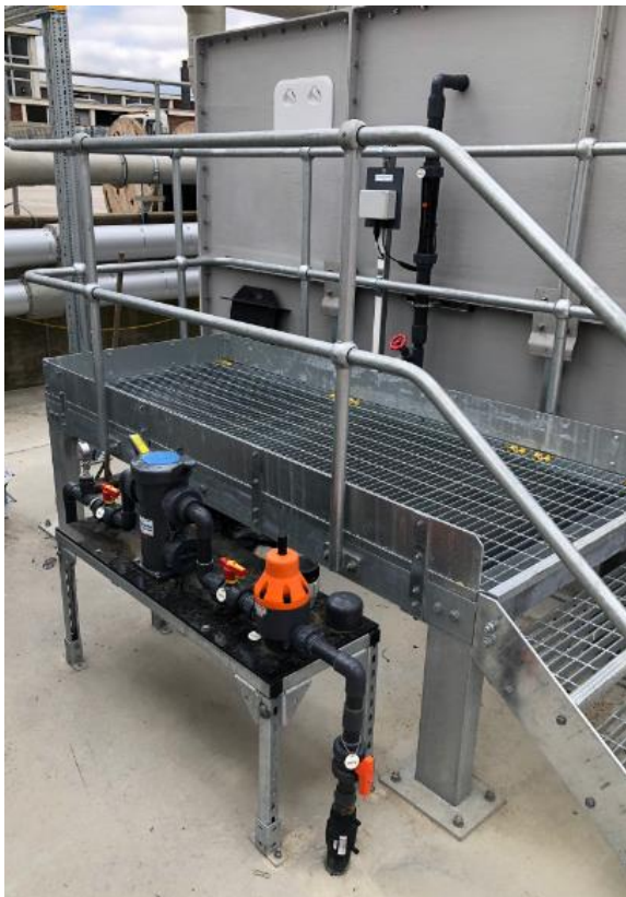
Biofilter irrigation (left) and high-level tank connection to odour control plant on slab (right)
