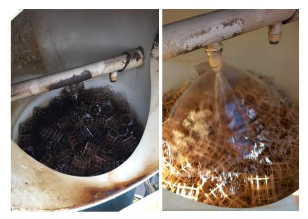
All the quench tower packing media was fully exposed to the caustic cleaning solution so coupled with the jet washing that MTS carried out we can be confident that the overall cleaning efficiency is as good as it could be.
