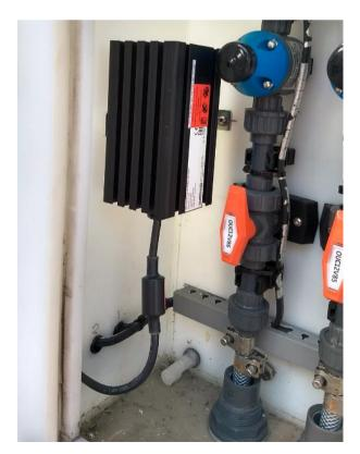
Integral cable routed out of enclosure via M20 IP68 stuffing gland (side wall of enclosure drilled and tapped to accept gland thread), through existing finger trunking containment up to trace heating power supply terminal box located at rear of caustic + hypo' POA enclosures.
