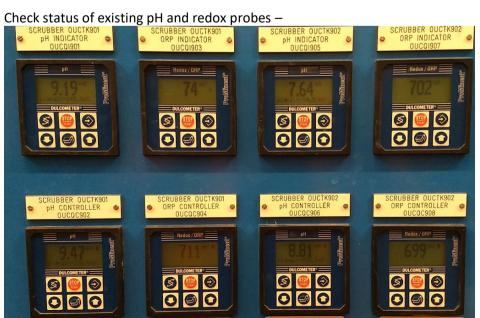
Scrubber #1 pH – two instruments showing 0.28pH difference, not ideal but not sufficient to inhibit automatic dosing.
